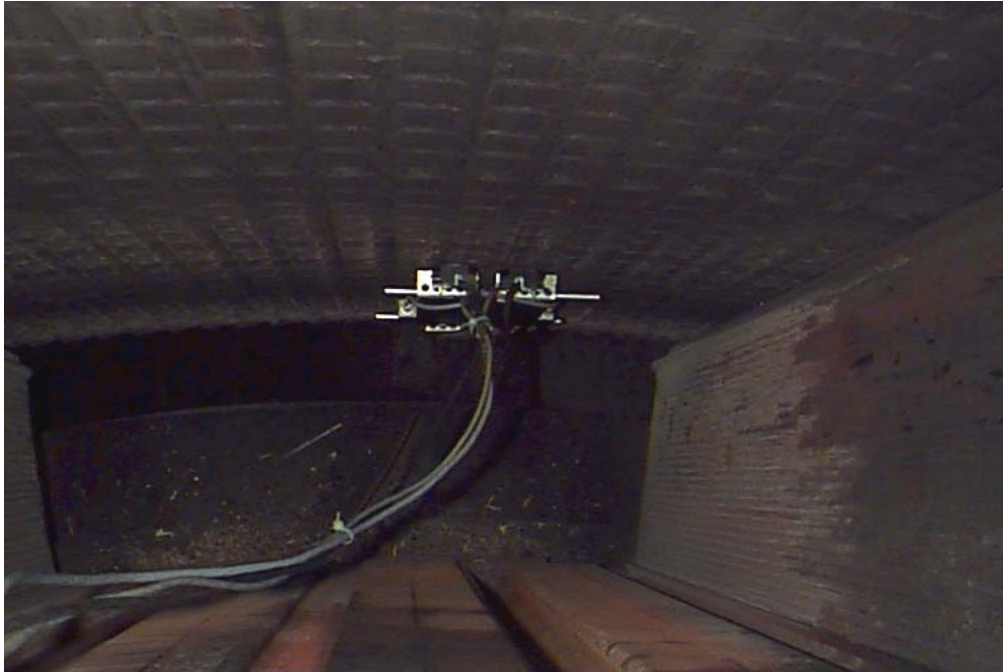
Figure 9. Robotic Vehicle with dual chattock coils traversing a single slot
